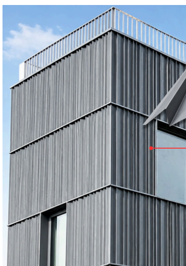
PANEL TYPE : W450U Rib height 45-79 mm. wide 450 mm.
