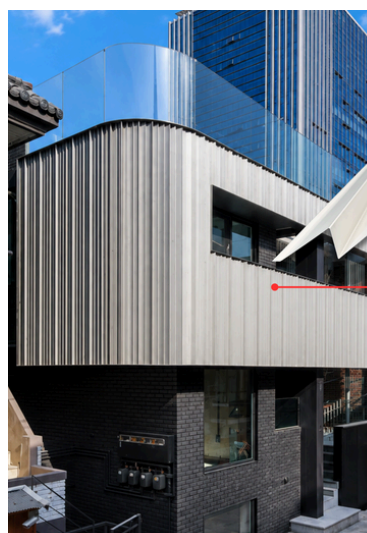
PANEL TYPE : W450T Rib height 60 mm. wide 450 mm.
