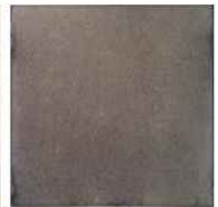
ZINCALUME® steel (No Sign of Rust)
